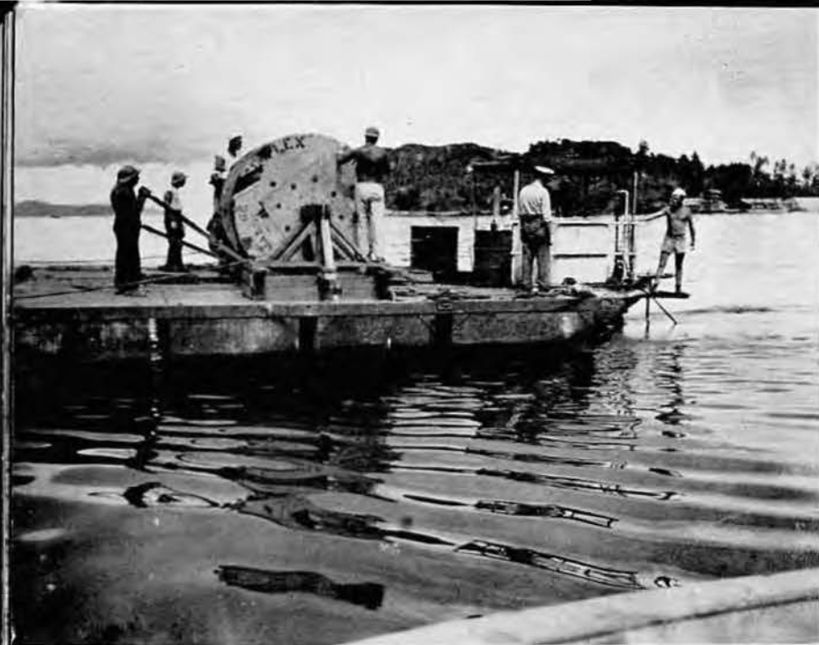
LAYING COMMUNICATIONS CABLE TULAGI
