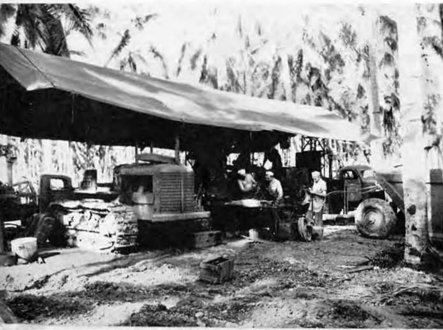
HEAVY EQUIPMENT REPAIR
