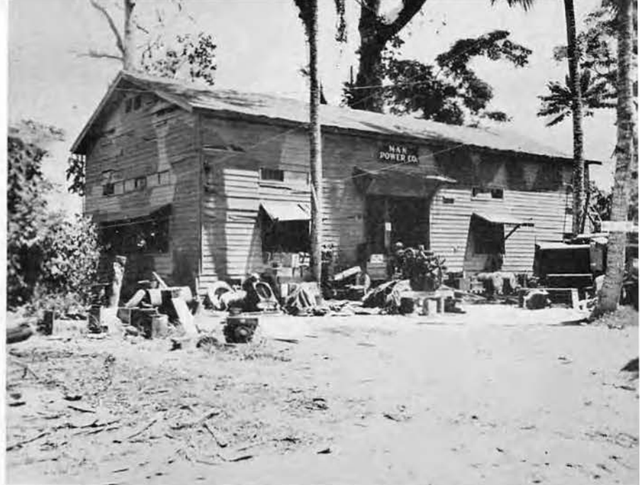
CAPTURED JAP POWER HOUSE
