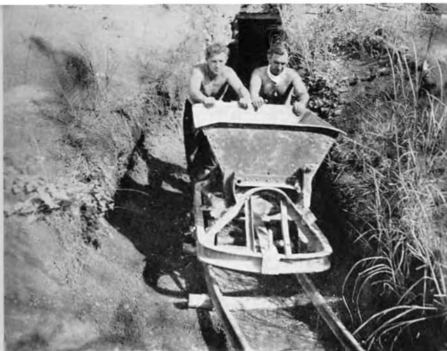
TUNNEL CONSTRUCTION USING JAP EQUIPMENT
