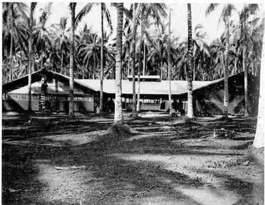
ISLAND RECREATION BUILDING
