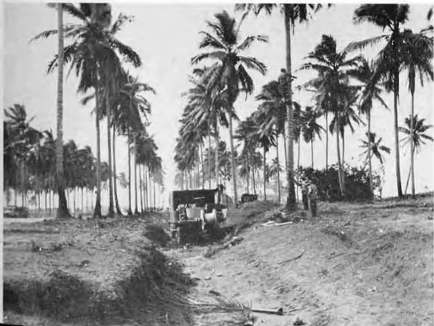
THE LINE CREW IN ACTION
